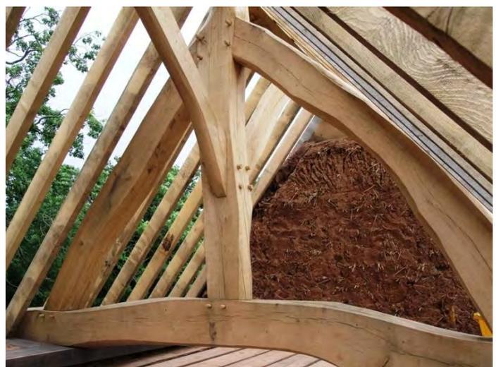
material which helps to bind the clay dabbin mixture together and regulate the rate at which it dries out. In clay dabbin construction straw not only goes into the mix but it is also laid independently on top of the clay layer, again helping to bind the layers while absorbing some of the moisture from the mix. This method of construction can be seen below.
