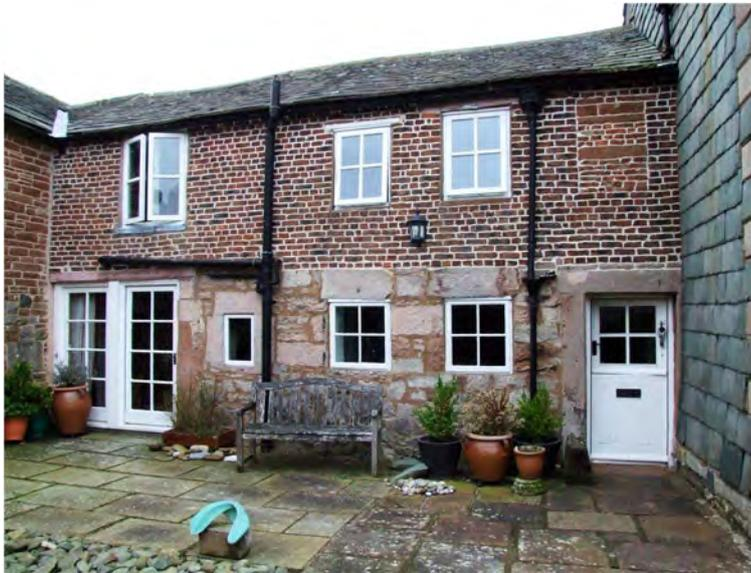
When the main block of the house was built in 1765, it was a partial rebuild. A section of the building to the left of the main block, remains from an earlier structure (left). It is one room deep in plan, and contains several features which are difficult to explain.
