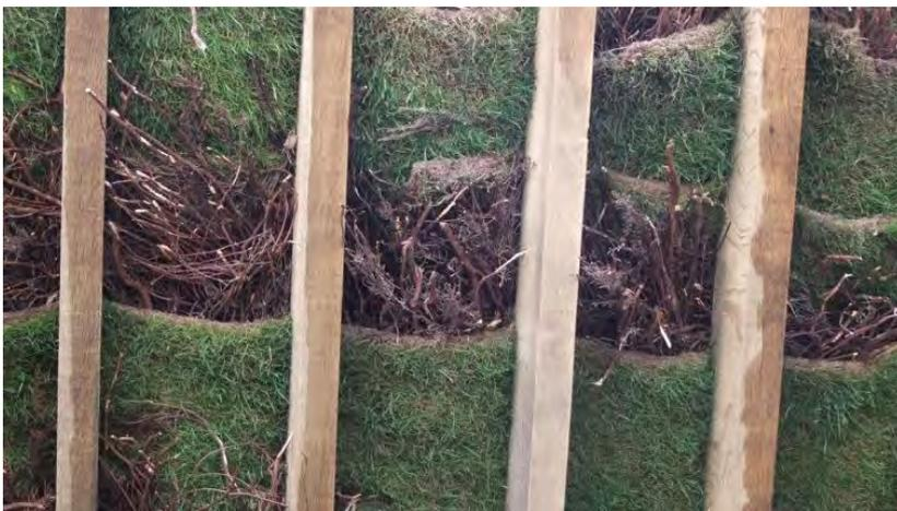
together and then pinned in place. Thatch itself can consist of a wide variety of vegetation including reed, straw (predominantly wheat but sometimes rye) and occasionally bracken. Reed normally has the longest lifespan, bracken the shortest. Today local derived thatch is rare. This example of heather
